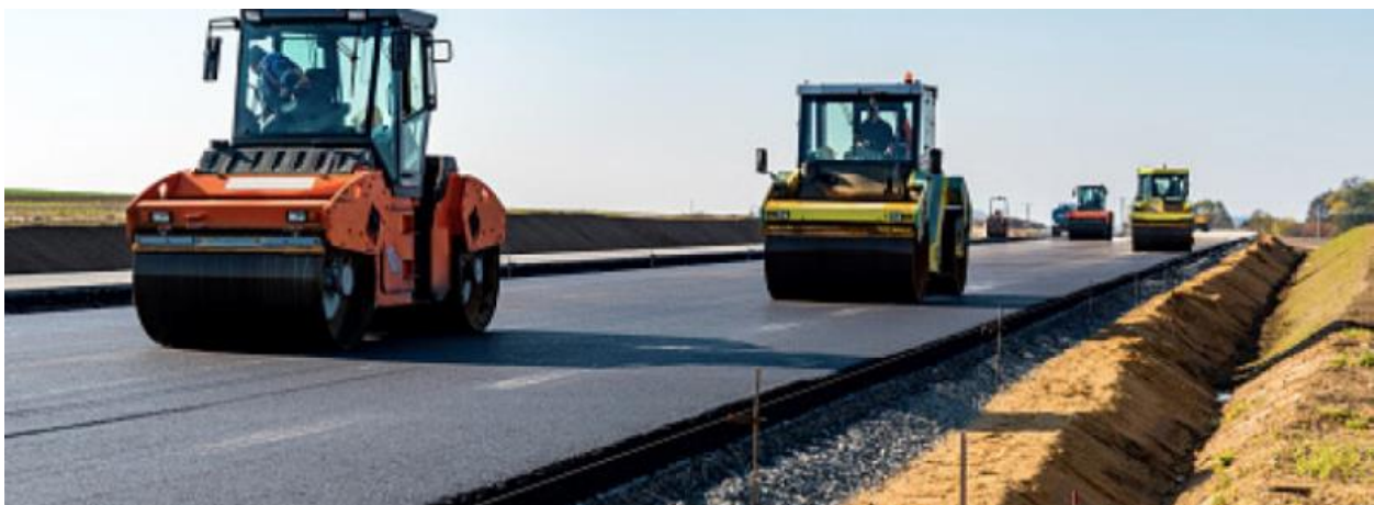
Figure 2. Rubber modified asphalt road. Source: Liberty Tire Recycling
